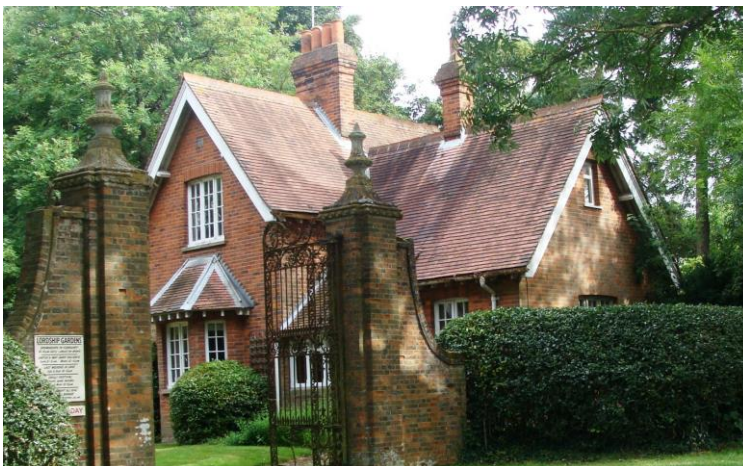
Picture 11. The Lodge an ancillary listed building to Benington Lordship probably dating from the early 20th century.
