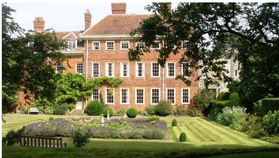
Pictures 6 and 7. Benington Lordship a fine grade II* listed building with 7 window range to south elevation and a tall Norman revival gatehouse with twin flint-faced circular towers to north east.
