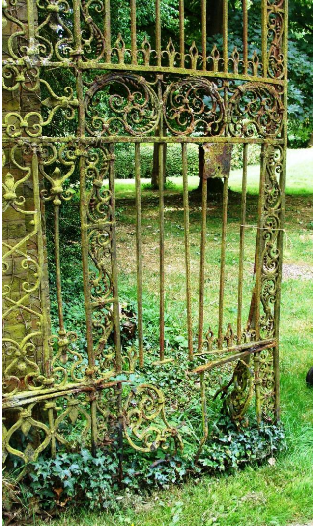
Picture 19. Fine entrance gates to Benington Lordship in urgent need of repair.
