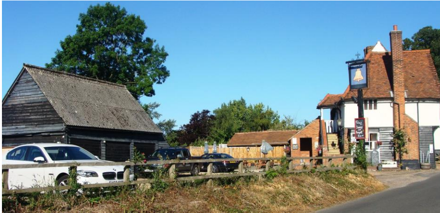
Picture 36. The exposed nature of the Bell PH car park will be much improved once the hedge to front has matured. Possible further improvements could be sought by some small number of strategically located tree planting. Note: since this photograph was taken the asbestos outbuilding in the picture is currently being refurbished.
