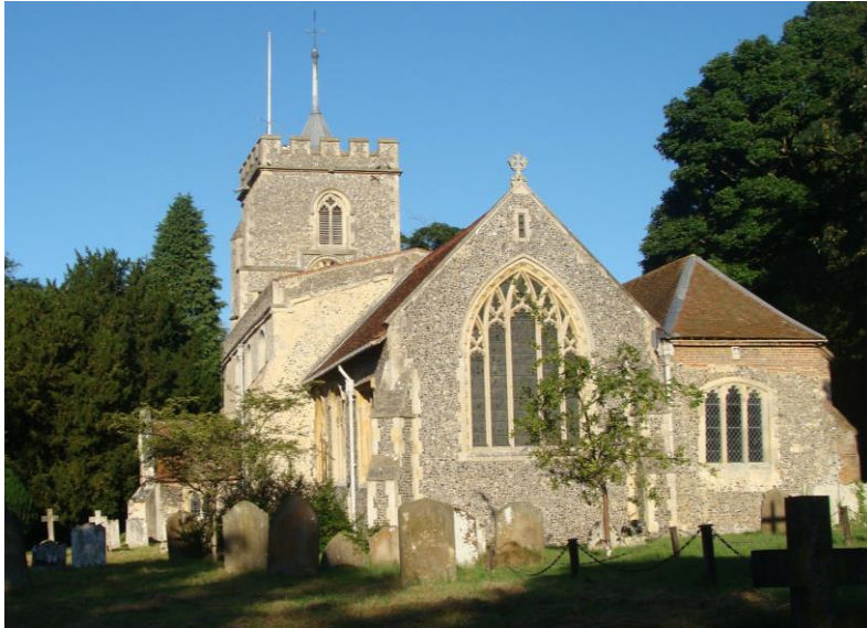
Picture 3. Grade I church of St. Peter occupies a prominent elevated location in the conservation area.
